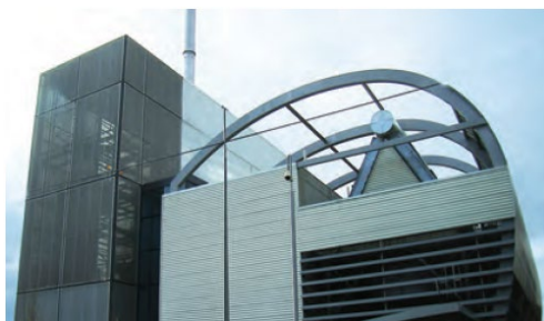
An innovative design to an Energy from Waste facility in an urban setting (Chineham, Hampshire).
