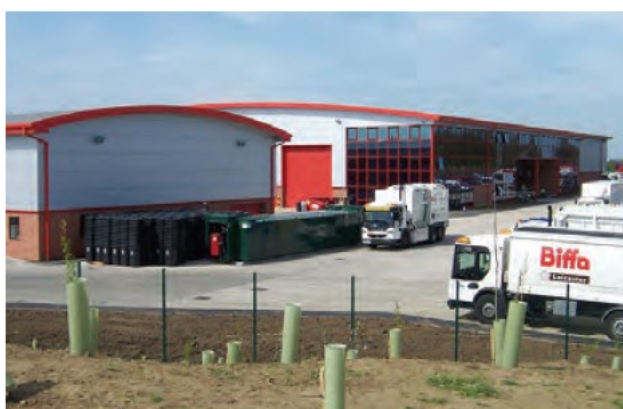
Leicester MBT 'Ball Mill' Site, an example of how a site can be kept clean and litter free through appropriate storage and fencing.
