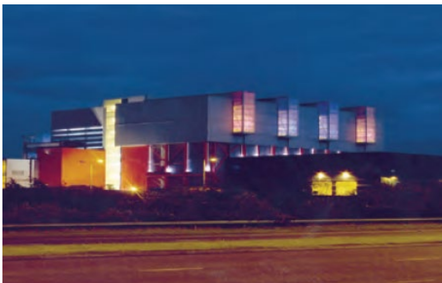
In urban areas a bold lighting scheme which enhances the building could be considered, such as this facility in Tyseley, Birmingham.
