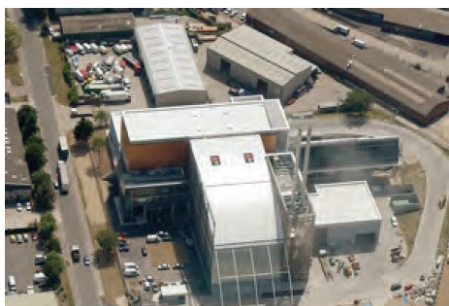
Portsmouth Energy Recovery Facility, which has a successful street frontage with its operational areas sited to the rear of the plot.
