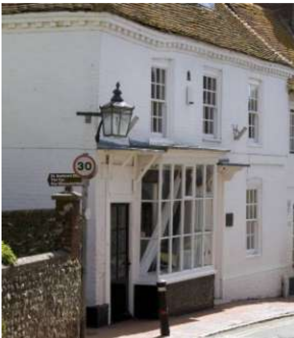
Fig. 7. The Old Paint Shop, High Street.
