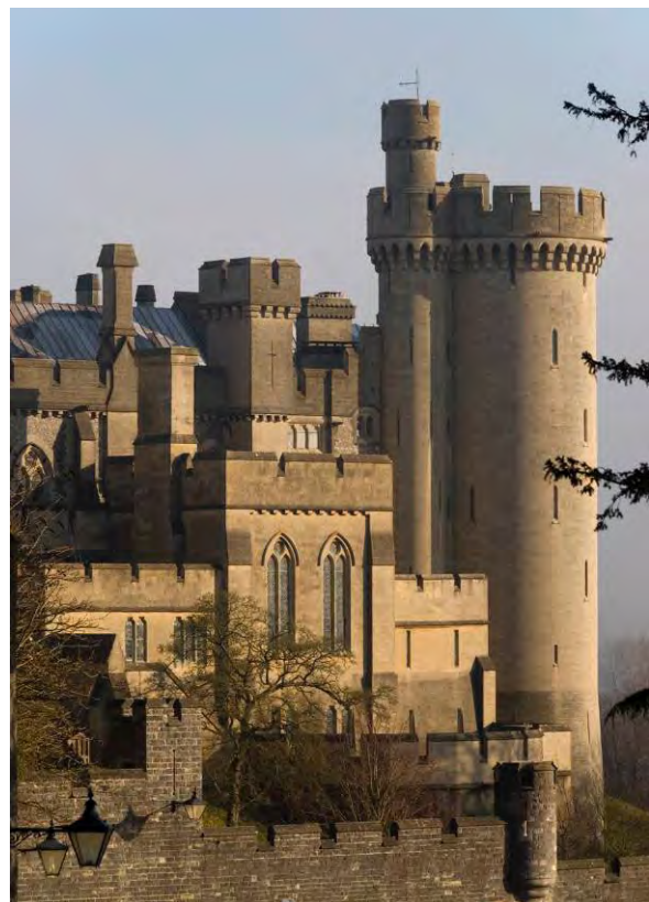
Fig. 28. Arundel castle: south-west tower from the west.
