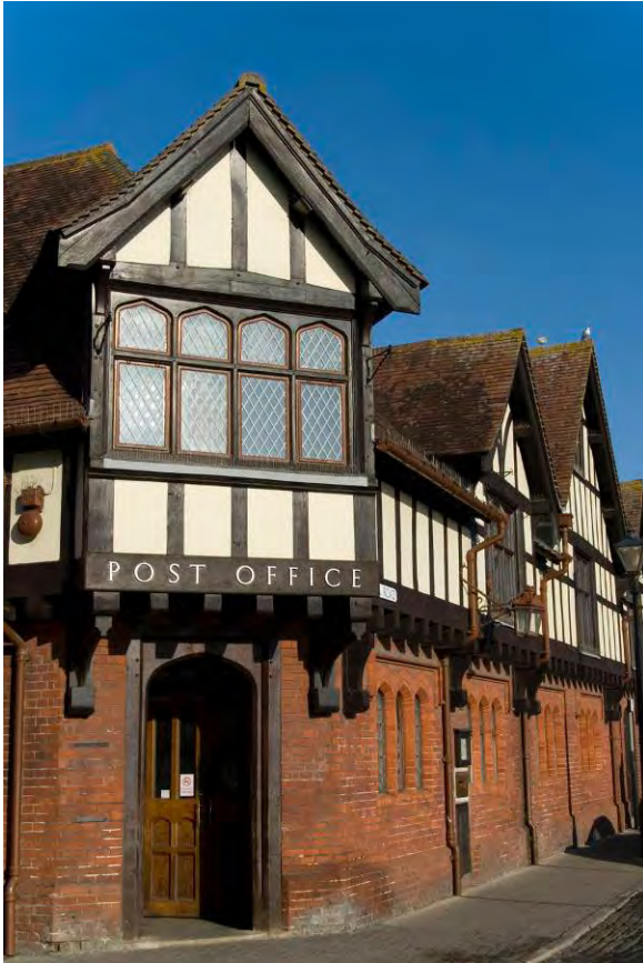
Fig. 29. Post Office, 2-8 High Street.
