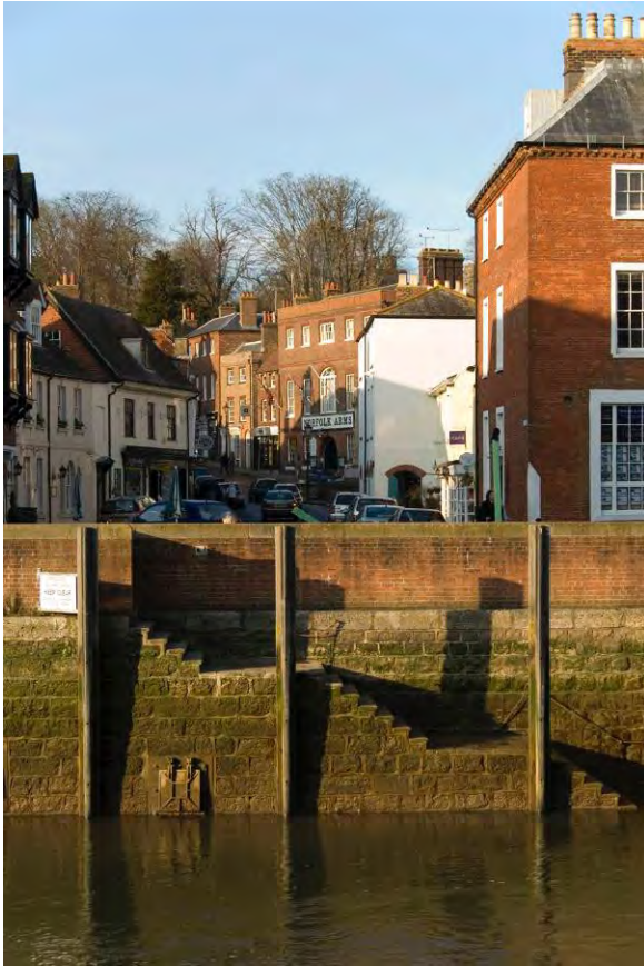
Fig. 2. View northwards across the River Arun to the High Street.
