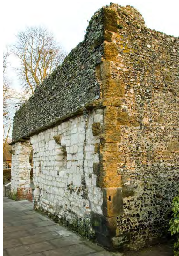
Fig. 19. Blackfriars: view of north side of south range of the conventual buildings, showing former cloister abutment.
