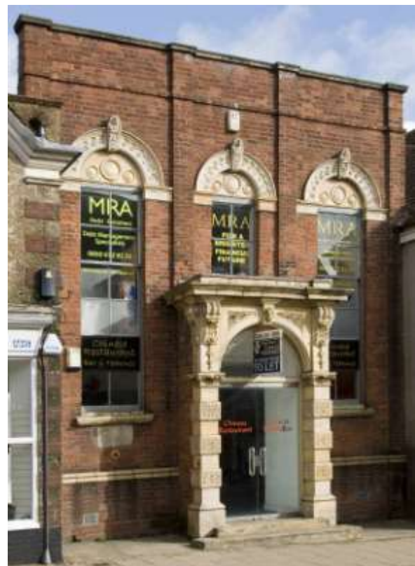
Fig. 30. Former Congregational (later United Reformed) church, High Street.
