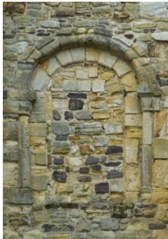
Fig. 14. Gatehouse: first-floor west window.
