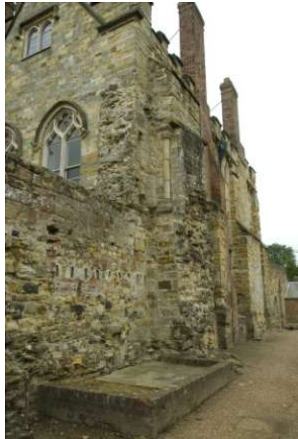
Fig. 13. South-west corner of nave of abbey church.
