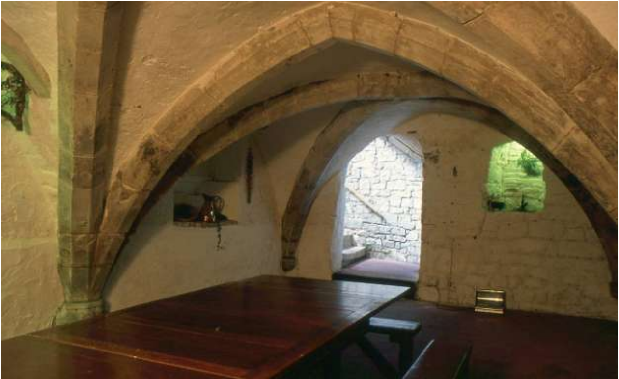
Fig. 22. 33-5 High Street: undercroft looking southwards. 178
