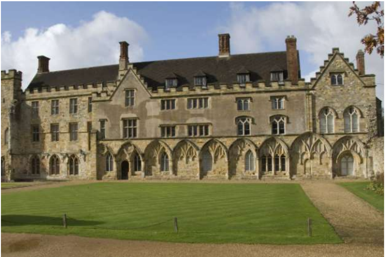
Fig. 16. Abbot's lodging from the east, showing west wall of cloister.
