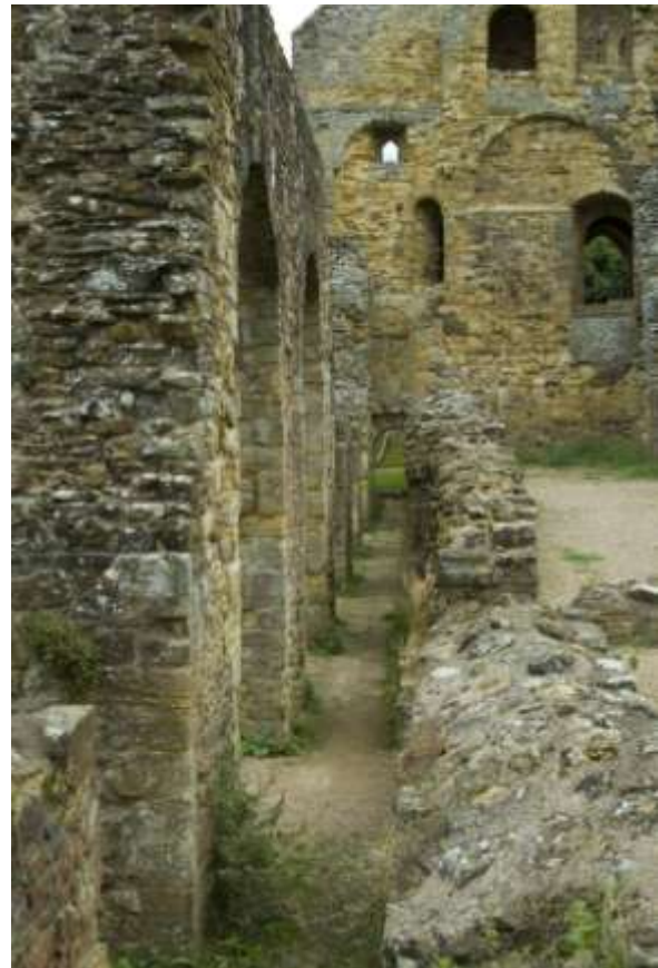
Fig. 19. Reredorter: view west along drain.
