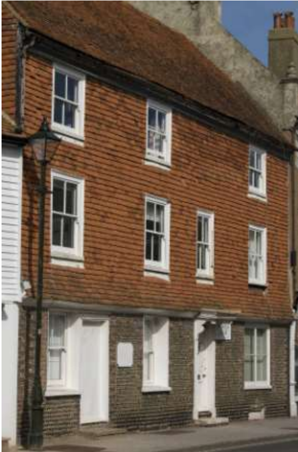
Fig. 15. Boswell House, 22 High Street: 18 th -century façade to possible earlier house.
