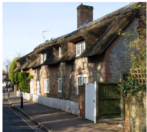
Fig. 16. Vicarage, Boniface and Primrose Cottages, Bersted Street, South Bersted.
