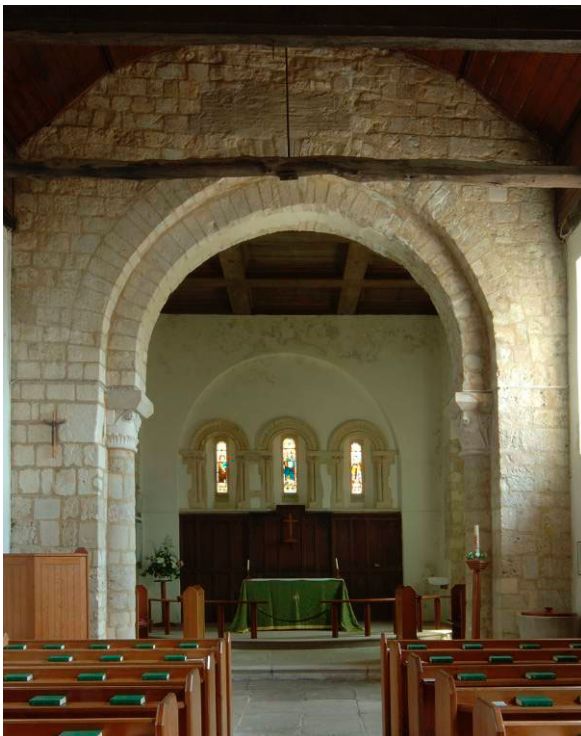
Fig. 9. St Nicholas's church: late 11 th -century nave from the west.
