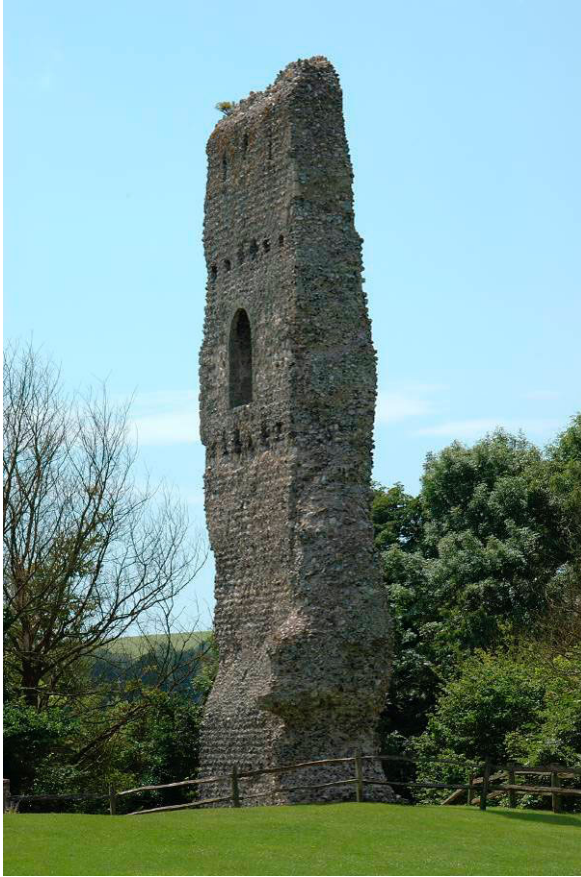
Fig. 7. Bramber castle gatehouse-keep: surviving west wall.
