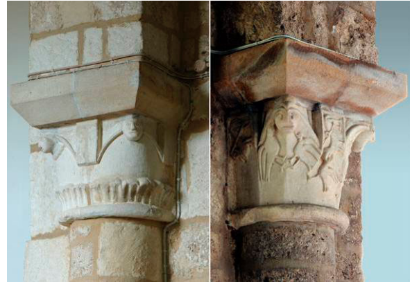
Fig. 10. St Nicholas's church: volute capitals of nave arch of (former) crossing. Left, northern respond; right, southern respond.
