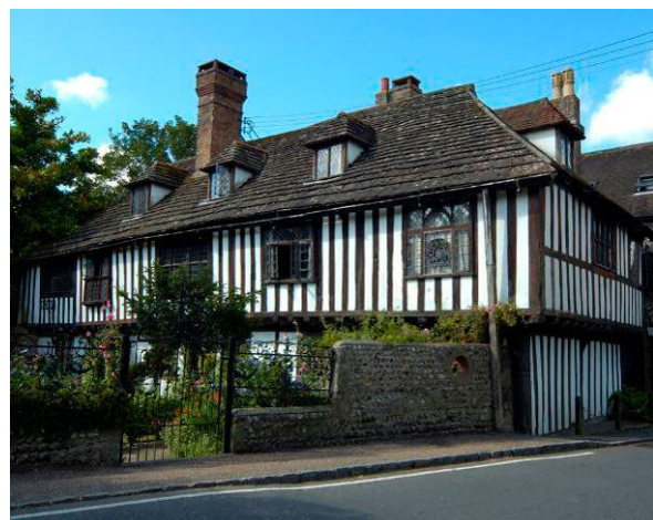
Fig. 12. St Mary's: 15 th -century timber framing.
