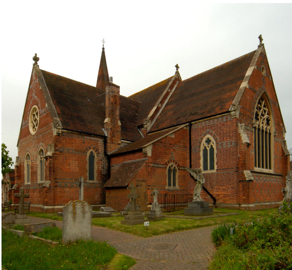
Fig. 9. St John's church from the south-east.
