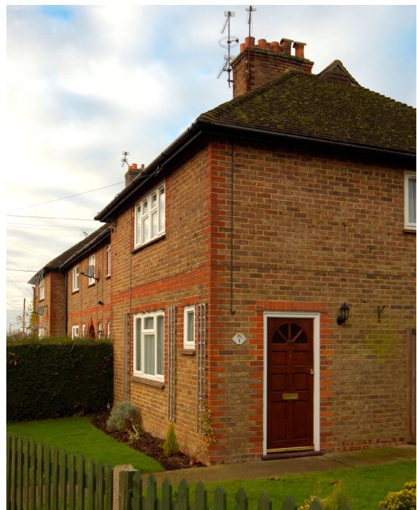
Fig. 13. Inter-war council housing at Norman Road.
