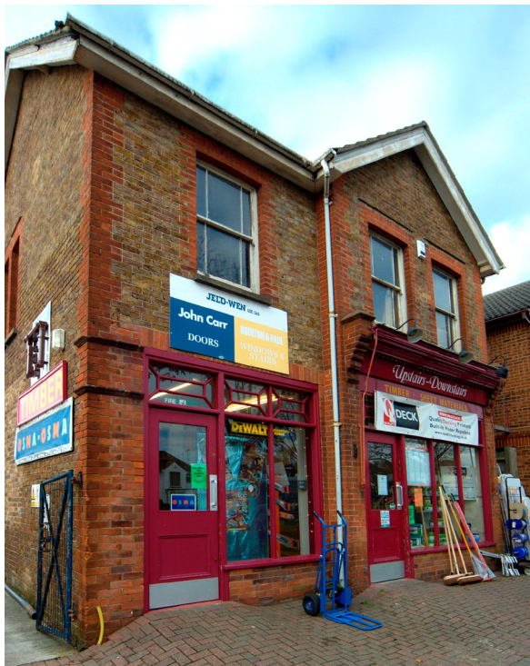
Fig. 4. Edwardian purpose-built shop at 133 London Road.
