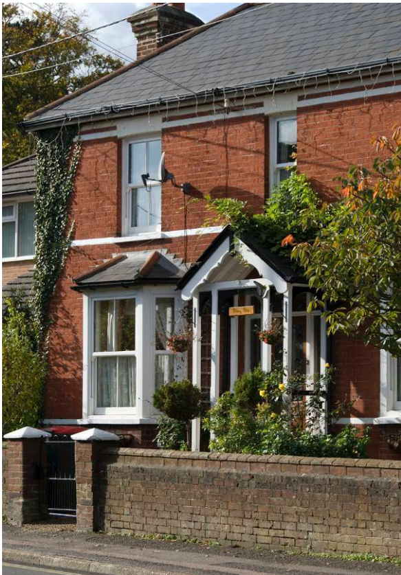
Fig. 6. Albany Villa, 25 Horsham Road: late 19 th -century detached villa.
