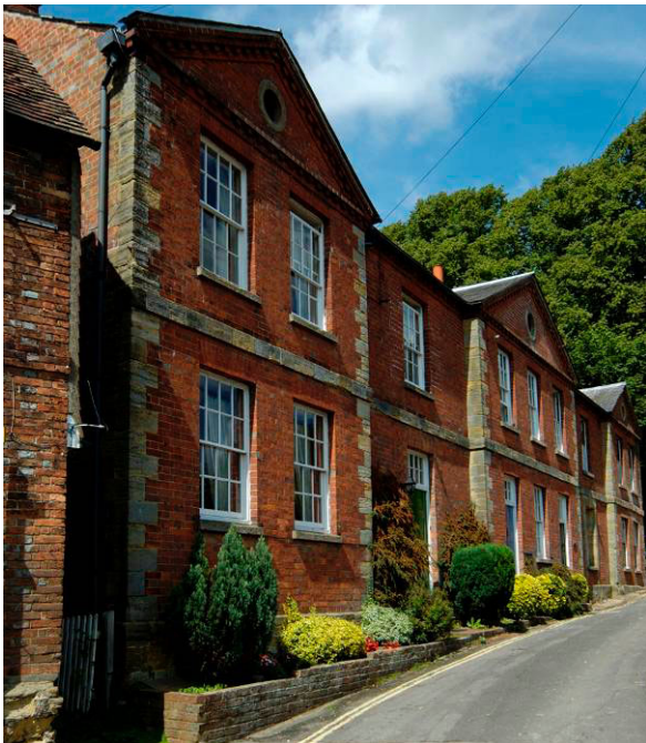
Fig. 9. The former workhouse, Ockenden Lane.
