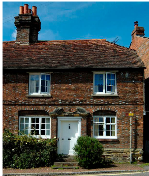
Fig. 15. 22 South Street: façade of 1722 to 17 th -century timber-framed house.
