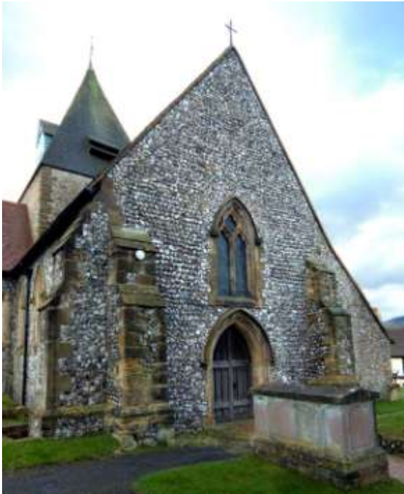
Fig. 10. St Margaret's church: west wall of nave.
