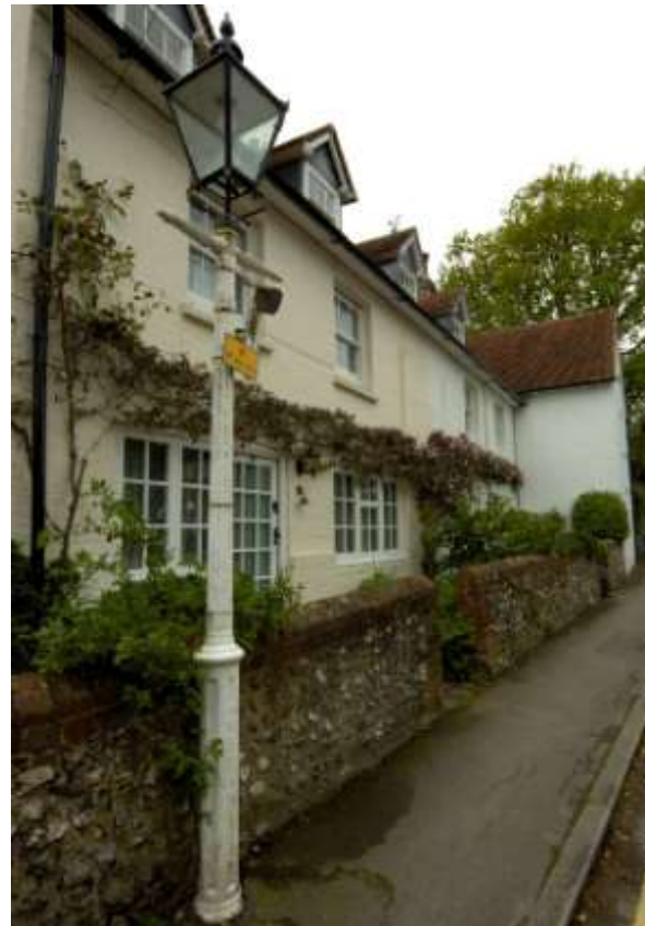
Fig. 9. Former Baptist free school, 28-32 East End Lane.
