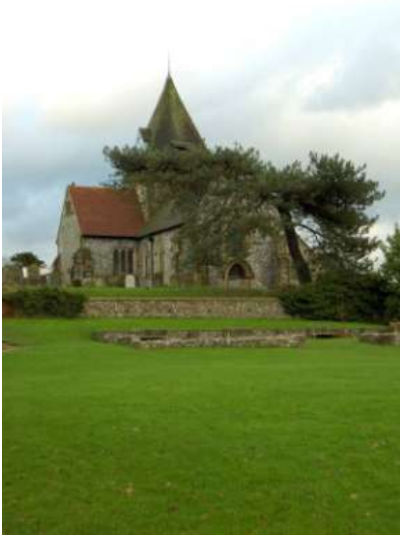
Fig. 3. St Margaret's church from the west, with the remains of Court Farm in the foreground.
