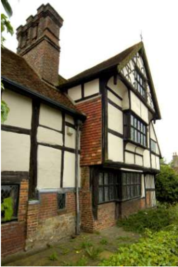
Fig. 14. Wings Place, 24 West Street: 16 th -century timber framing.
