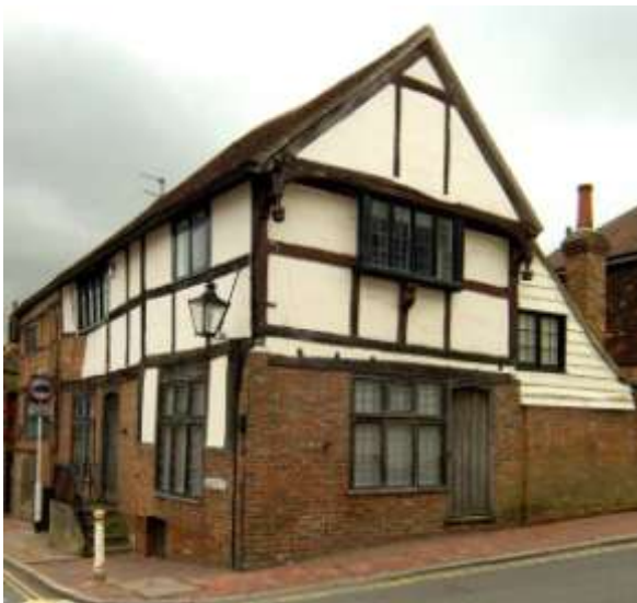
Fig. 15. 1 South Street, showing northern gable.
