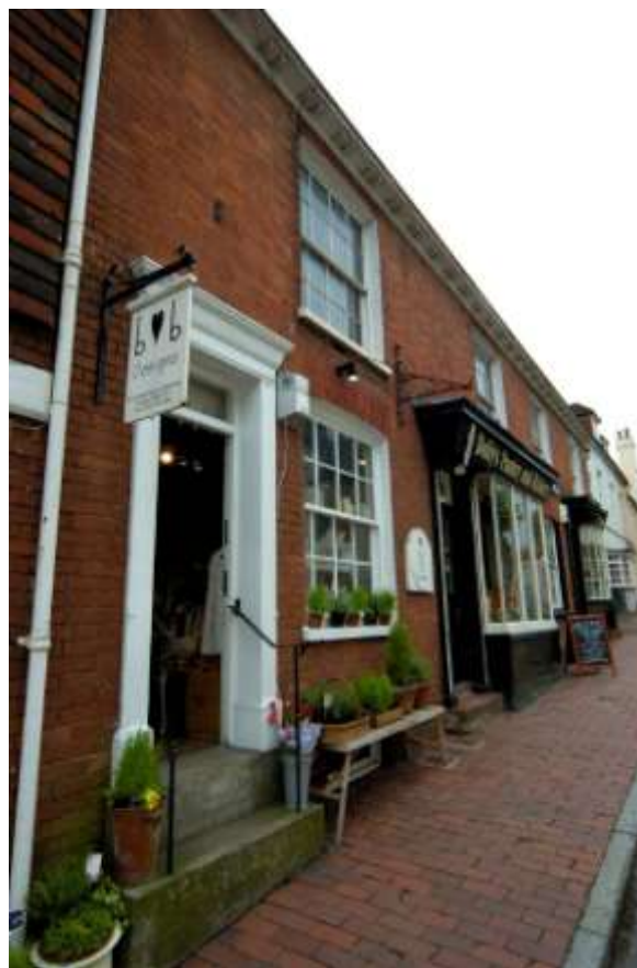
Fig. 8. Surviving shops at 19 th -century 4-8 West Street.
