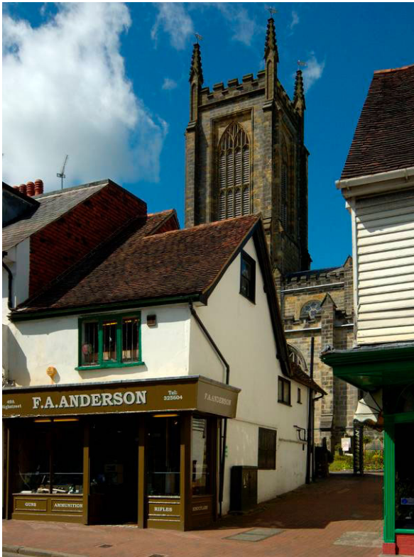
Fig. 4. High Street 'cottages' without substantial back plots, built in front of the churchyard.
