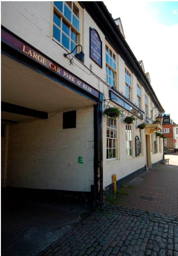
Fig. 5. The Dorset Arms, 58-62 High Street (formerly the Cat), refaced in brick in the early 18 th century.
