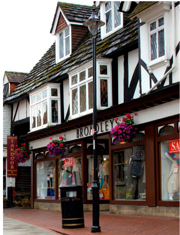
Fig. 12. 14 th -century timber framing at 34-40 High Street.
