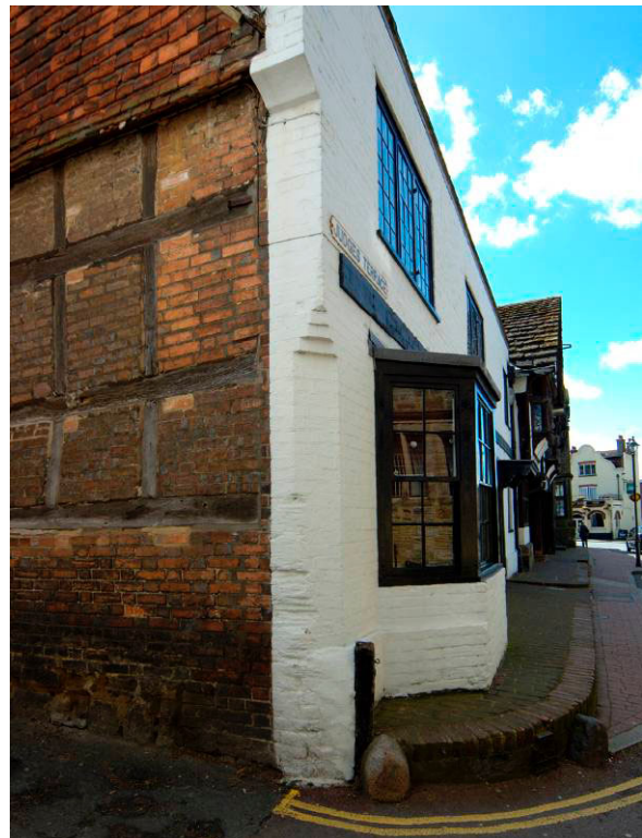
Fig. 15. 1-2 Judges Terrace, High Street: 18 th -century façade applied to mid-15 th -century timber framing.
