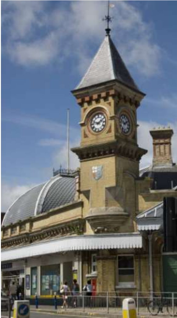
Fig. 10. Eastbourne railway station (as rebuilt 1886).
