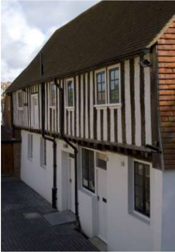
Fig. 26. Old Parsonage Barn: west elevation.
