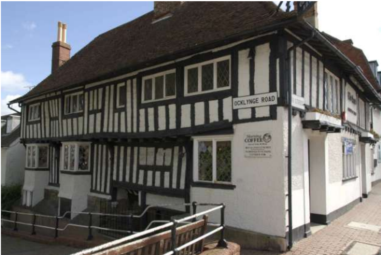
Fig. 4. The Lamb Inn: a much modified Wealden house, with an earlier undercroft (see section 4.1.1).
