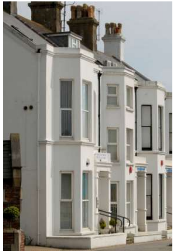
Fig. 18. 30-6 North Street: late 19 th -century housing.
