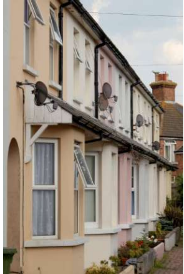
Fig. 6. Terminus Place: terraced housing by the station (c.1900).
