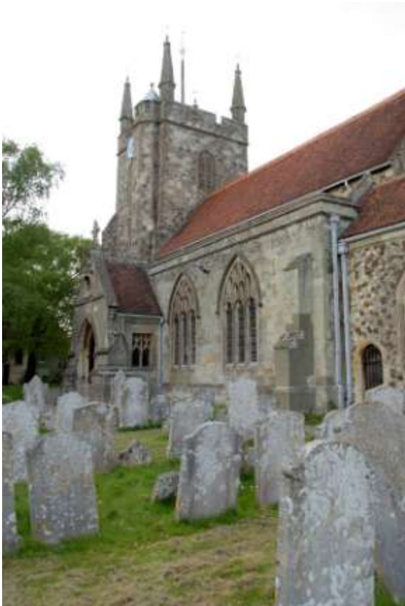
Fig. 3. St Mary's church from the south-east.
