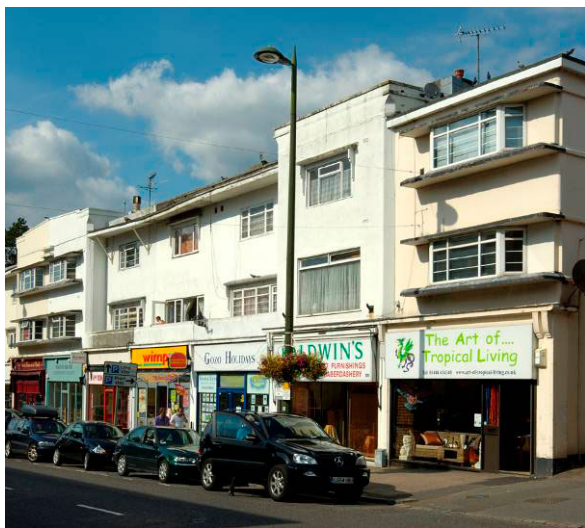
Fig. 11. Pre-war shops and flats, 118-20 South Road.
