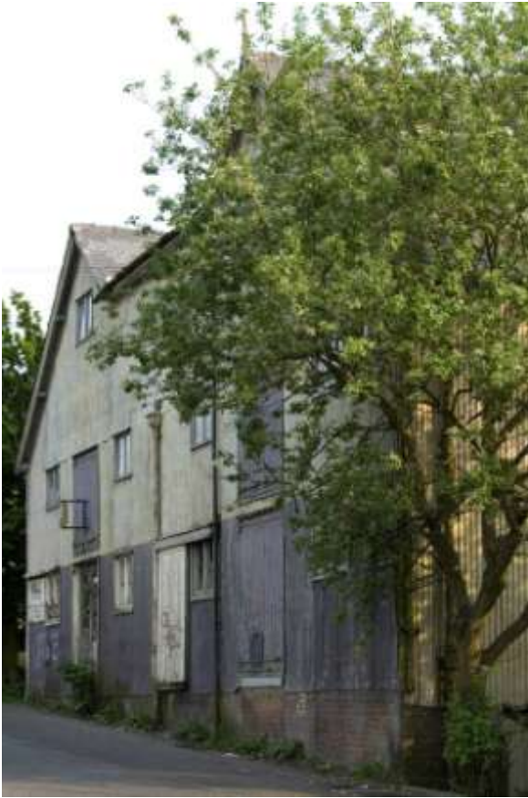
Fig. 6. Corn mill, Station Road (disused).
