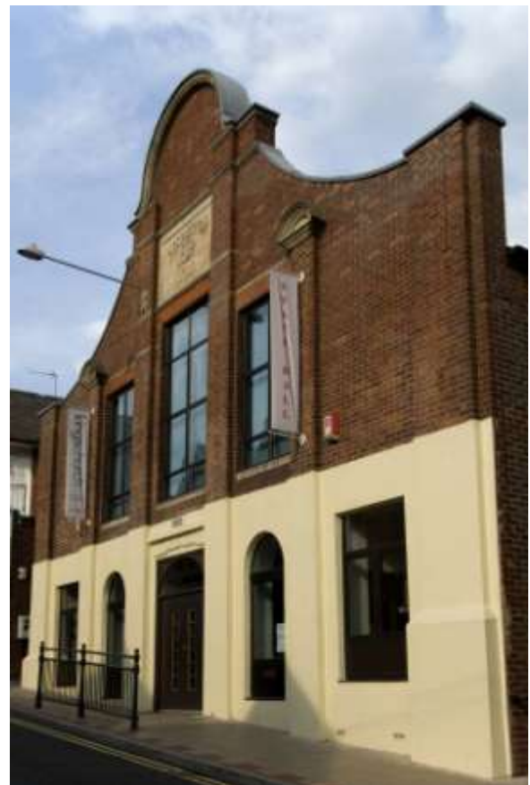
Fig. 9. The State Hall, Station Road.
