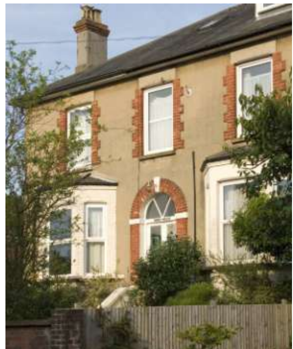
Fig. 16. Late 19 th -century Derby House, Hailsham Road.
