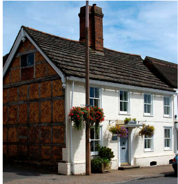
Fig. 15. Greenfield House, High Street: 17 th -century timber framing with 18 th -century brick façade.
