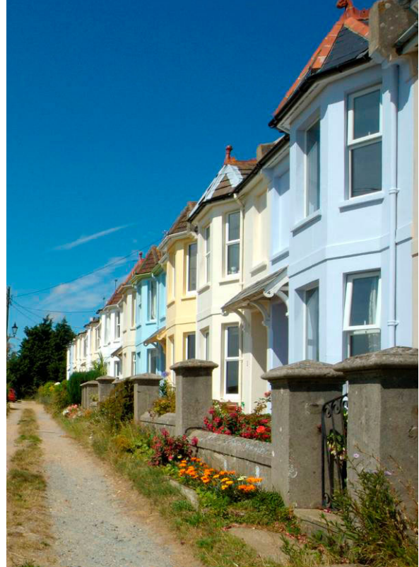
Fig. 20. Southview Terrace, Nep Town. Bay windows and stucco of railway age housing (c.1880).
