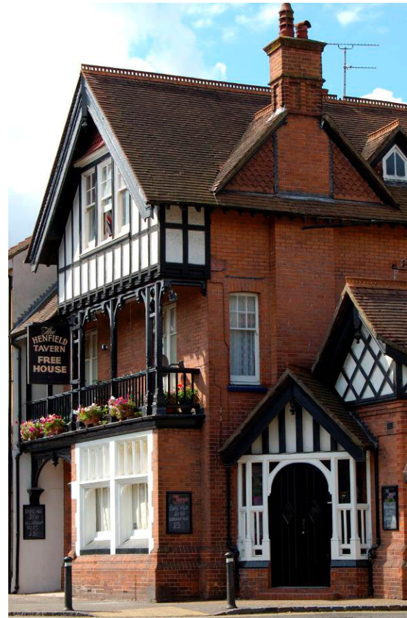
Fig. 18. Henfield Tavern, High Street. Edwardian vernacular revival.
