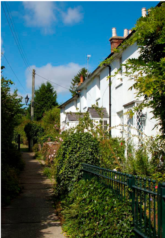
Fig. 11. Church Terrace: probable encroachment on the churchyard.
