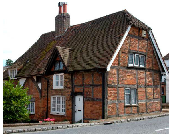
Fig. 13. Ganders, Golden Square. Late 14 th or early 15 th -century timber frame, with 17 th -century extension towards the street.
