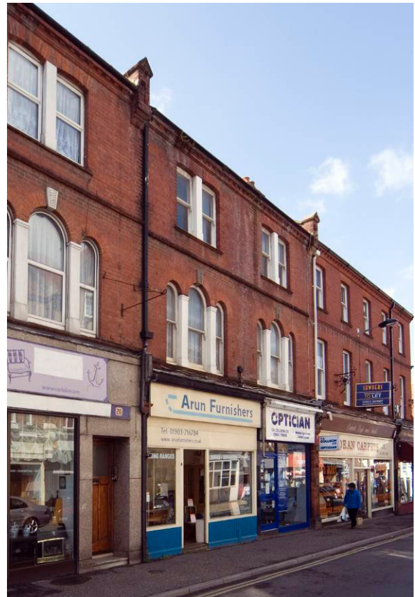
Fig. 27. Purpose-built shops at the north end of Beach Road.
