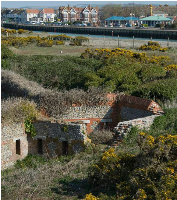
Fig. 13. Littlehampton fort: carnot wall and SE bastion.
