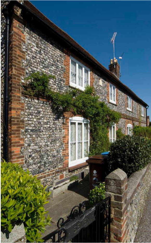
Fig. 19. Hampton Cottage, 7-9 Church Street.
