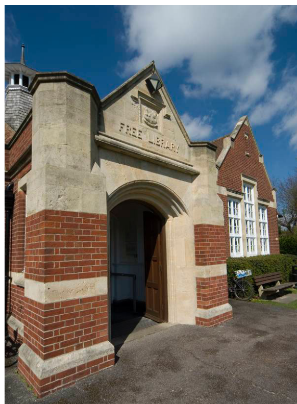
Fig. 16. Public library, Fitzalan Road.
