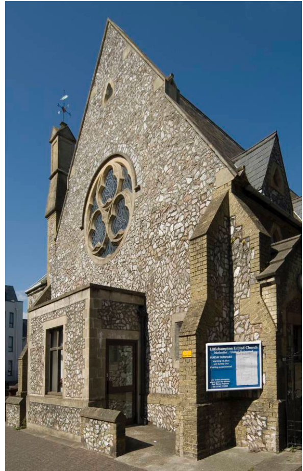
Fig. 12. Congregational church (now United Church), High Street.
