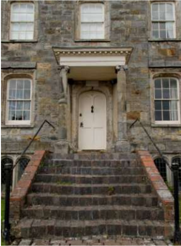
Fig. 19. The Stone House, High Street.
