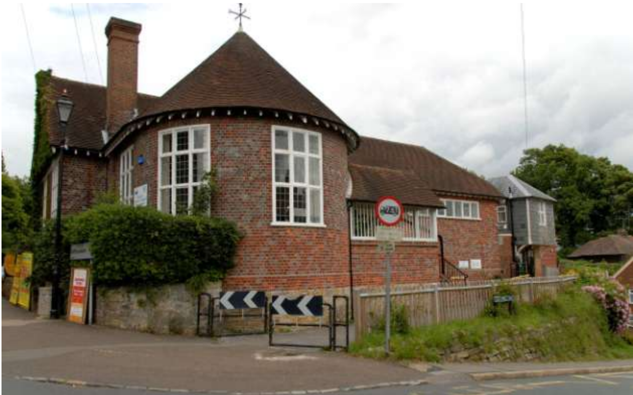
Fig. 9. Mayfield Church of England Primary School, largely as rebuilt in 1913.
