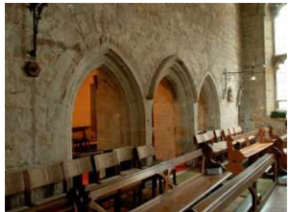
Fig. 11. Mayfield Palace: triple service doorways to former hall.
