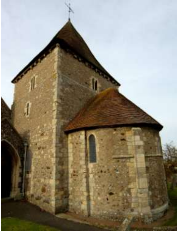
Fig. 11. St Michael's church: early to mid-12 th -century tower and apsidal chancel.
