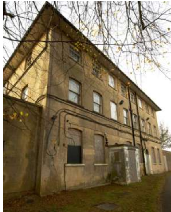
Fig. 13. Newhaven Union workhouse, Church Hill (1835).
