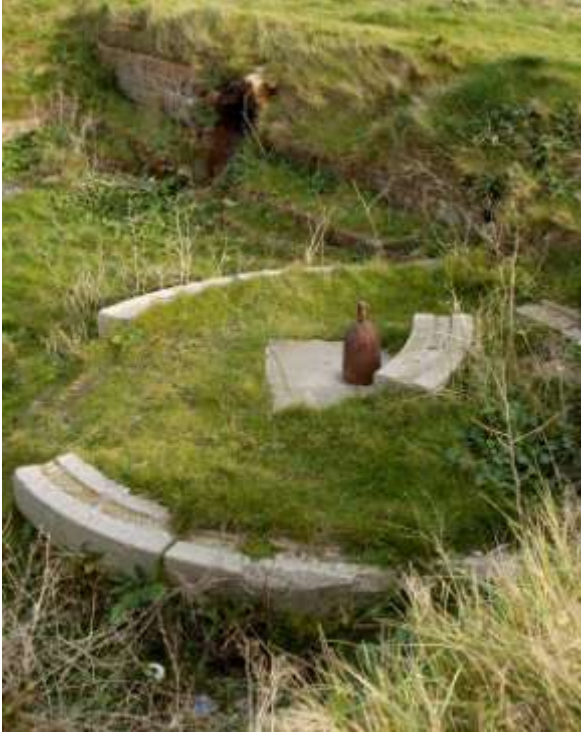
Fig. 18. Lunette Battery (early 1855), showing gun platform and, beyond, a magazine.
