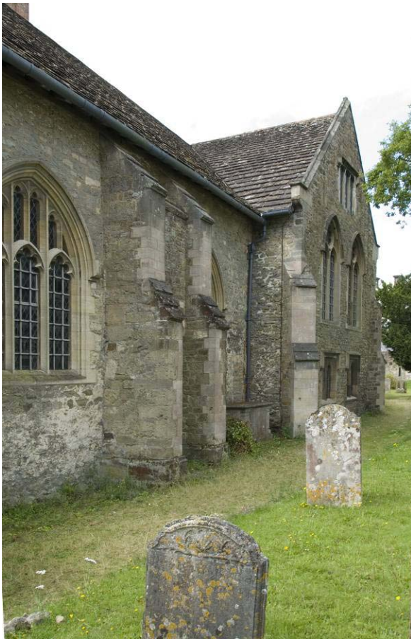
Fig. 10. St Mary's church: north elevation looking west showing north transept.
