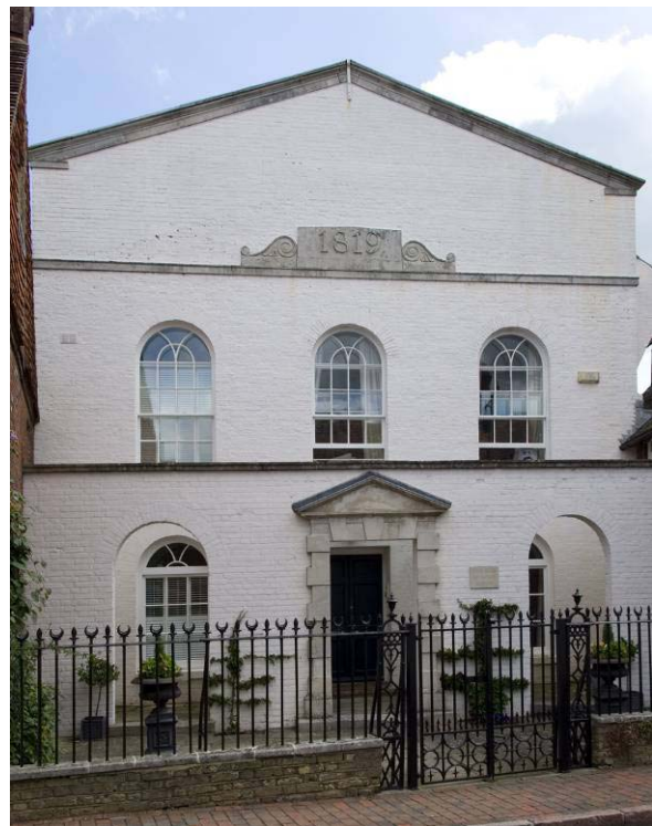
Fig. 6. Former Congregation chapel, East Street.
