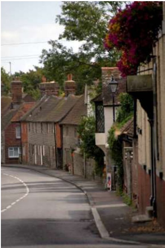
Fig. 12. High Street, south side: view east.
