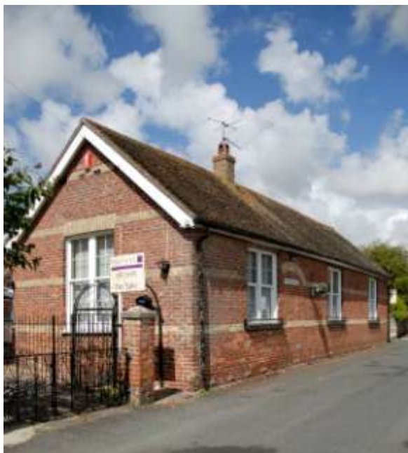
Fig. 9. Former National School (1876).
