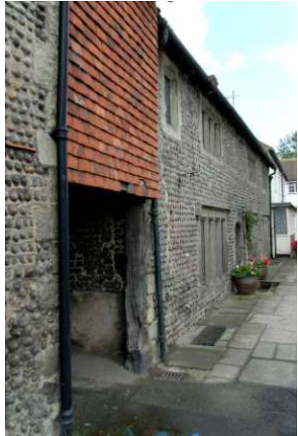
Fig. 14. Entrance to twitten by Penthouse Cottages.
