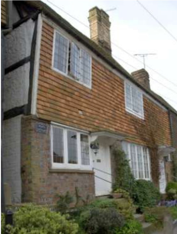
Fig. 11. 1-2 Chapel Cottages: 17 th -century timber framing visible in the end wall.
