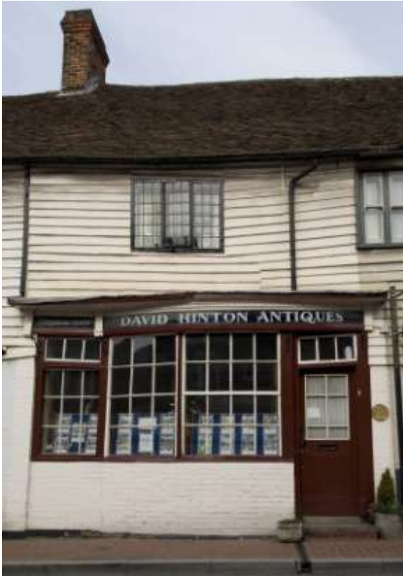
Fig. 6. Early 19 th -century shop front at 5 High Street.
