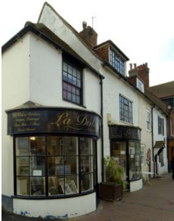
Fig. 11. 44-50 High Street. Behind the early 19 th -century No. 50 (foreground) is the gable of a timber-framed 17 th -century house, re-fronted with cobbles c.1800.
