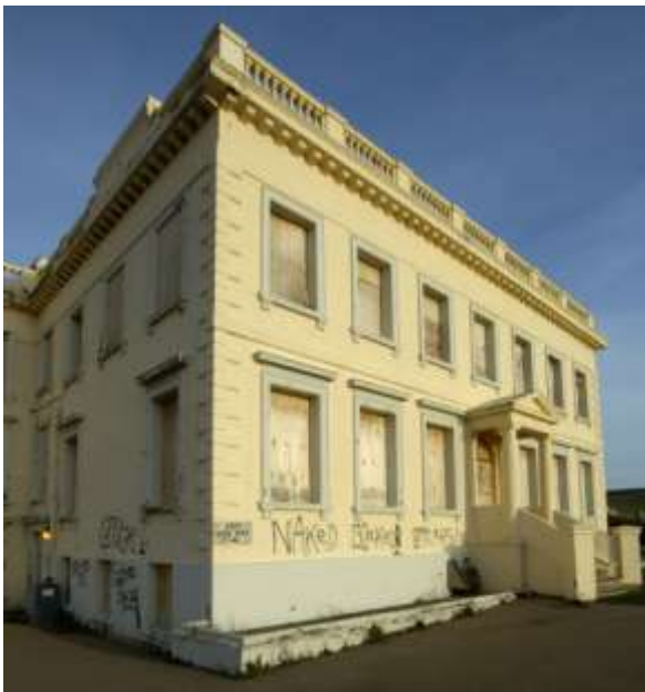
Fig. 13. Corsica Hall, south-west front.
