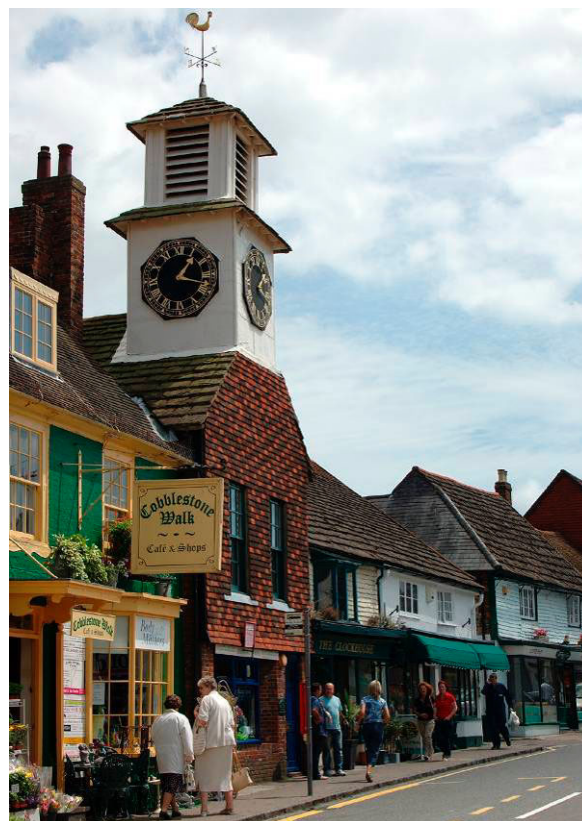
Fig. 5. Market House, High Street (1771).
