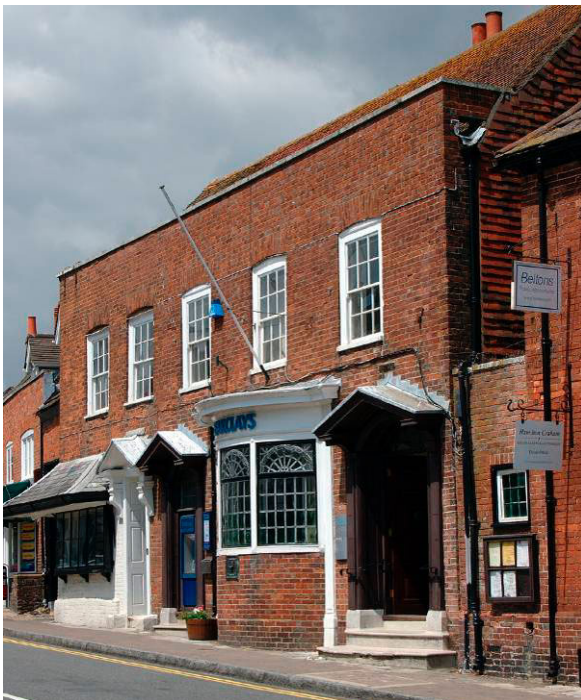
Fig. 10. 40-2 High Street: 18th-century rebuilding.
