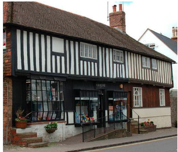
Fig. 9. 61-3 High Street: a continuous-jettied townhouse.
