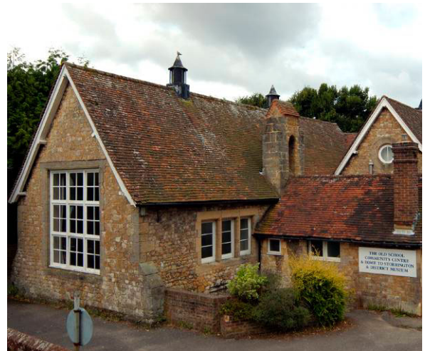
Fig. 16. The (former) school of 1868-73, School Lane.
