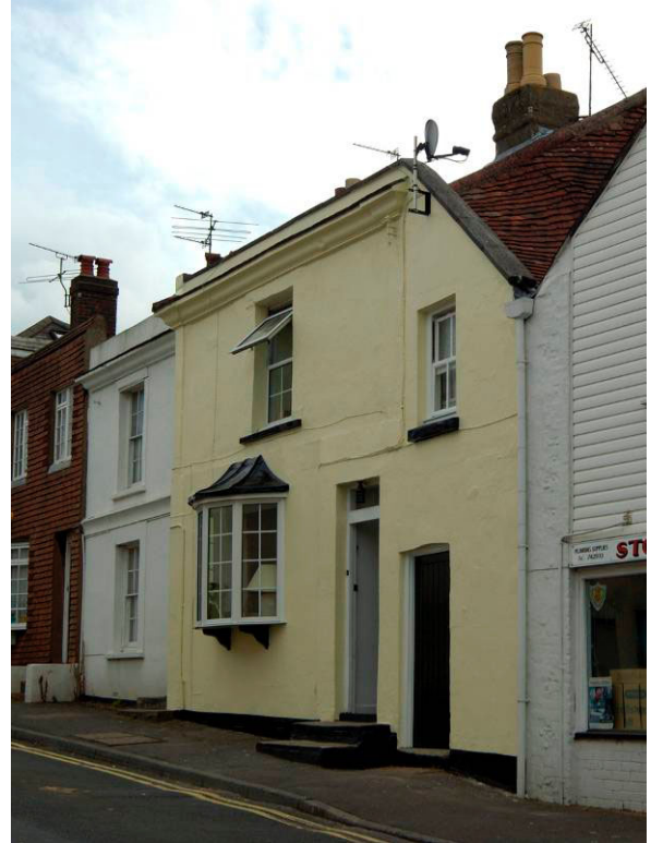
Fig. 15. The former Railway Inn, 14-16 School Hill.
