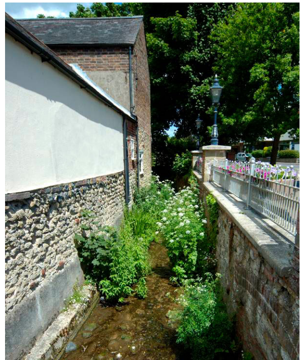
Fig. 6. The River Stor looking north from the High Street: Bine Mill was located on the right.
