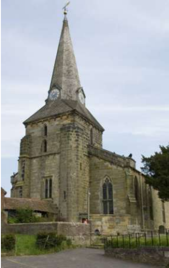
Fig. 4. Church of the Holy Cross, Church Street.
