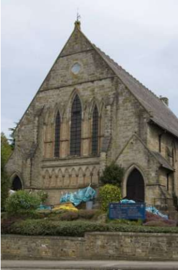
Fig. 9. Congregational chapel (now United Reformed Church), High Street, New Town.
