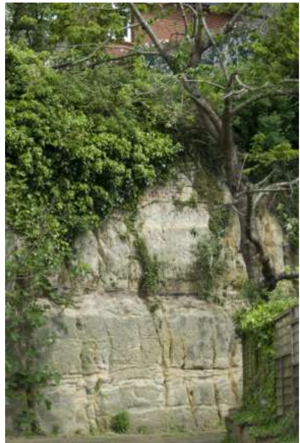
Fig. 3. Ardingly Sandstone exposed to the rear of 258-62 High Street.
