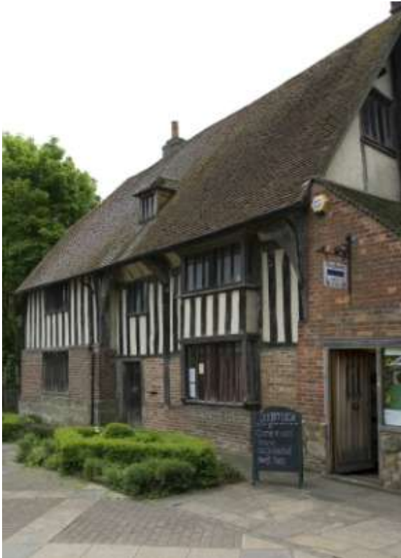
Fig. 13. Bridge Cottage, High Street.
