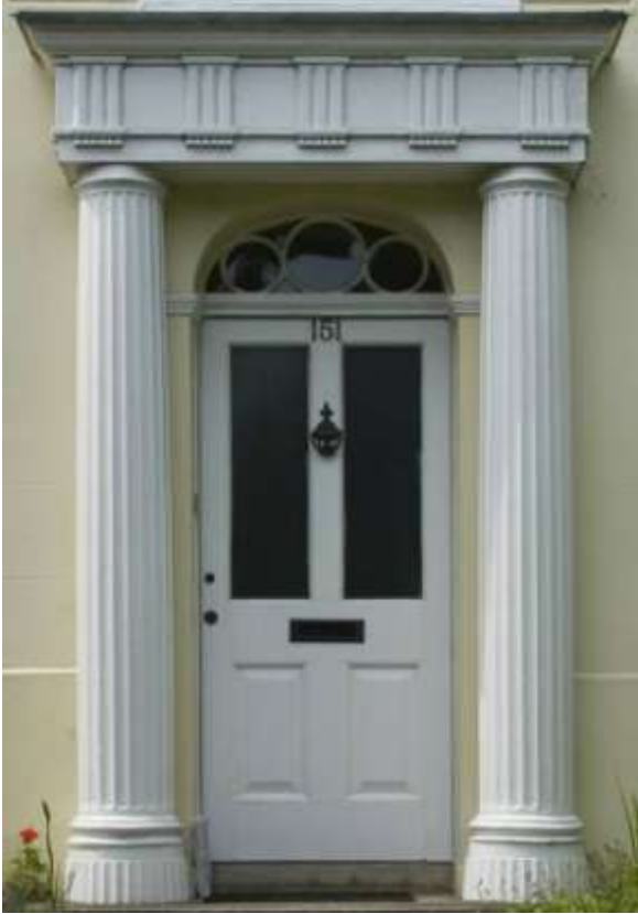
Fig. 20. 151 High Street: detail of front door.
