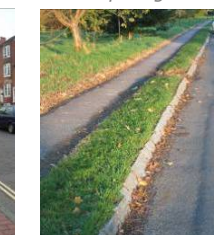
Rural angled kerb pavers
