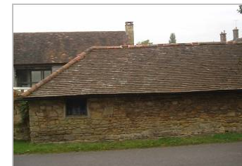
Stone farm out building
