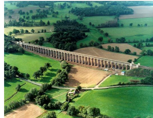
Ouse Valley Viaduct, 1841
