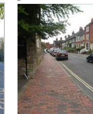
Red/multi brick pavers
