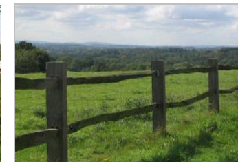
Hardwood post and rail fencing
