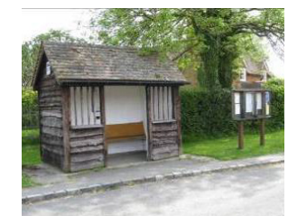
Timber bus shelter
