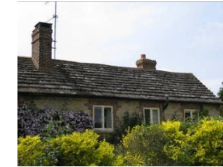
Horsham stone roof
