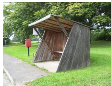
Contemporary timber bus shelter
