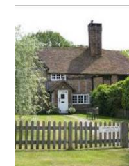
Timber framed house
