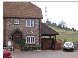
High quality social housing at Singleton using traditional materials and vernacular style
