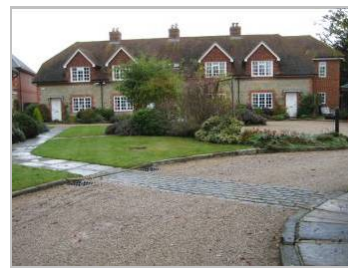
Recent development in Midhurst using locally distinctive materials
