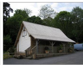
New village store at Lodsworth using locally produced materials including wood shingles
