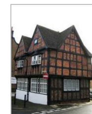
Brick & timber framing with brick nogging
