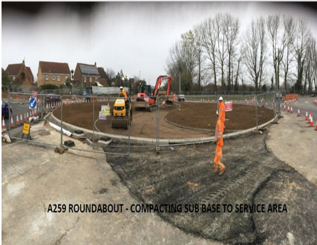
Figure 2: The A259 Worthing Road Littlehampton road improvements completed under a S278 Agreement
