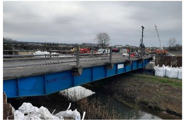
Figure 4: Temporary Bridge over Black Ditch
