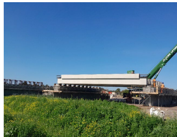
Image 5: The beams in position
