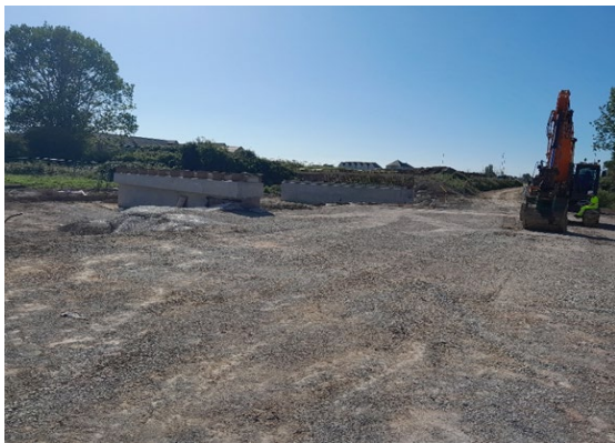
Image 6: Crane mat construction
