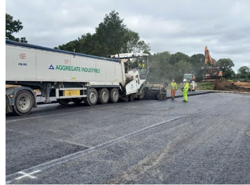
Image 3: Laying base course of surfacing
