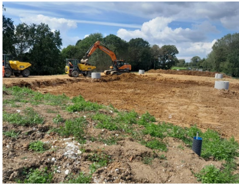
Image 1: Material being removed from the front of the surcharged to be placed further back.
