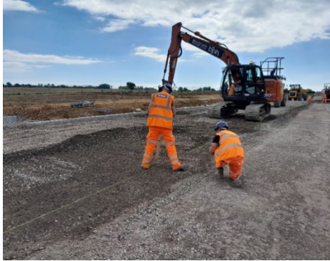
Image 2: Trimming the type 1 to level
