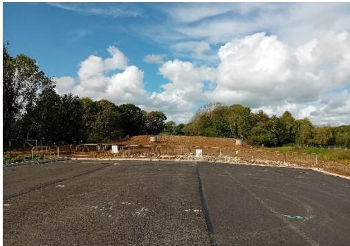
Image 2 Embankment with surcharge.
