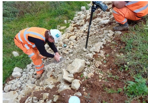
Image 1 Chalk sample taken for WAC testing.
