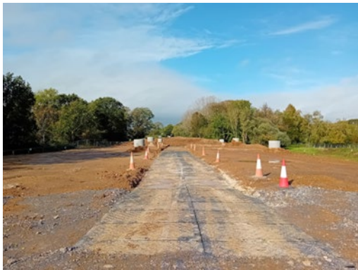
Image 1 Track mats placed running up to surcharge
