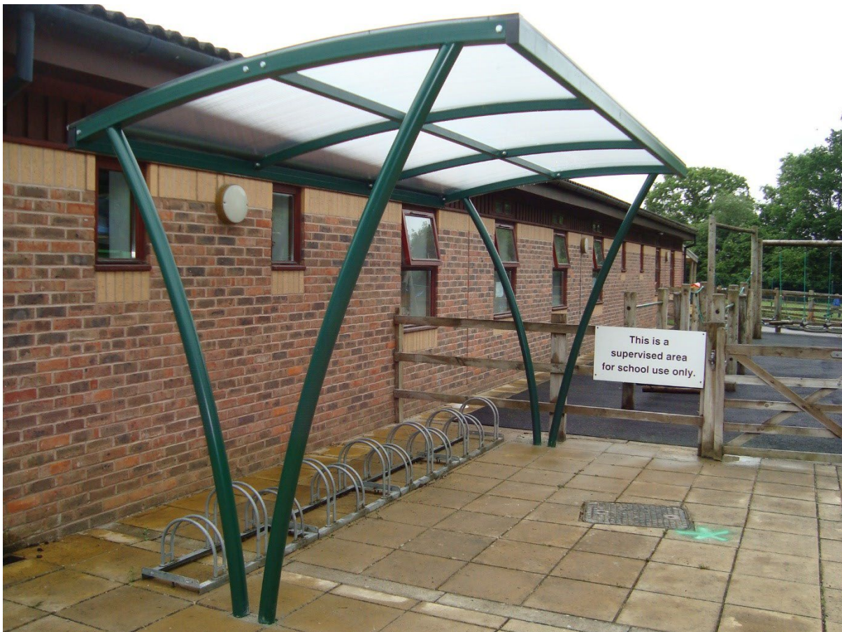
Castlewood Primary School Bike Shelters – implemented in 2020/21 using Highways S106 funds
