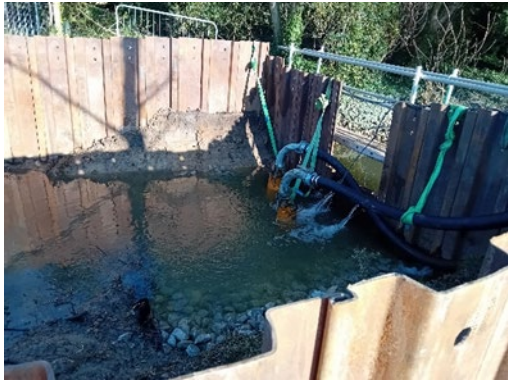
Image 1 Cofferdam with over pumping.
