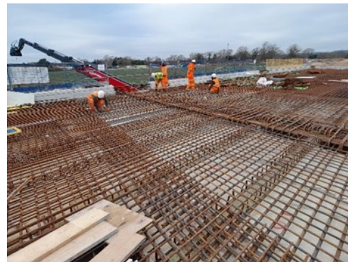
Image 6 Steel work progress
