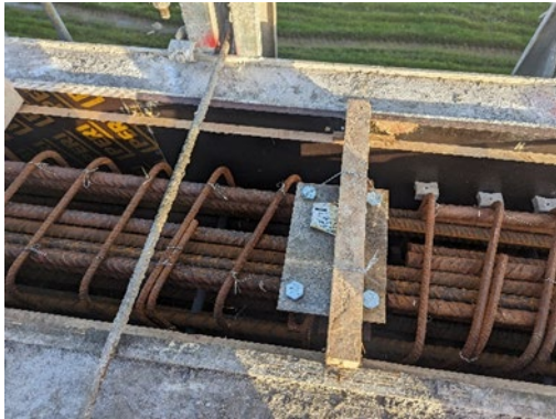
Image 7 Bolt cluster for parapet.
