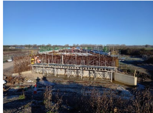
Image 8 View of viaduct facing North.
