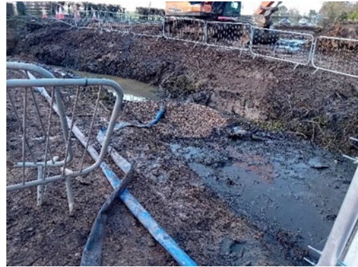
Image 2 location of new culvert.
