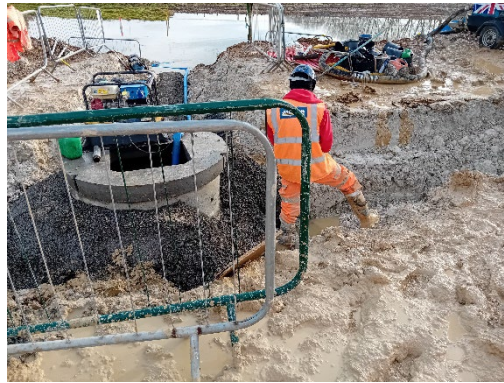
Image 3 Continued drainage works.
