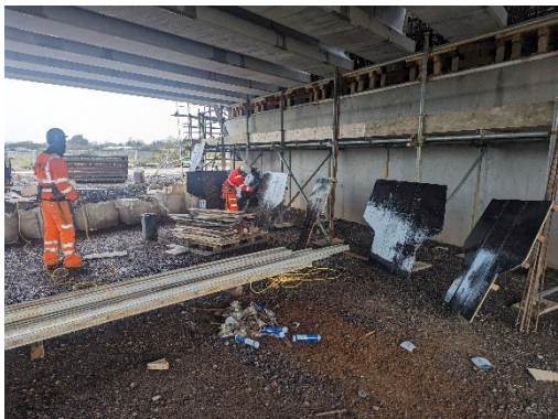
Image 8 Shutters ready for instalment.
