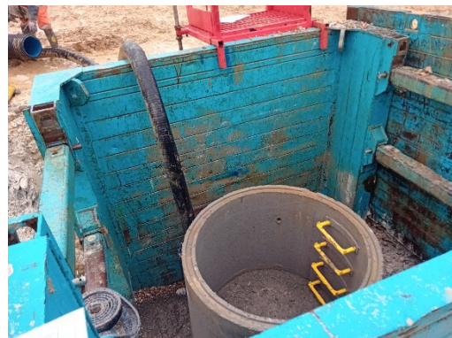
Image 2 Water pump in manhole trench box.
