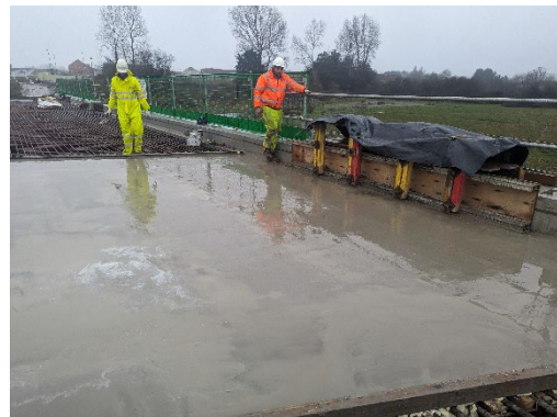
Image 9 Fresh concrete pour.
