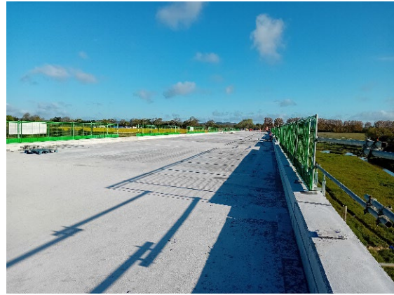
Image 7 Concrete deck by the end of viaduct
