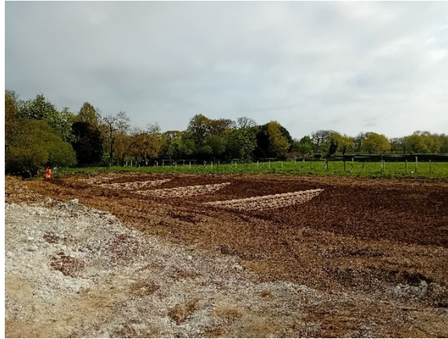
Image 3 Swale with concrete check dams
