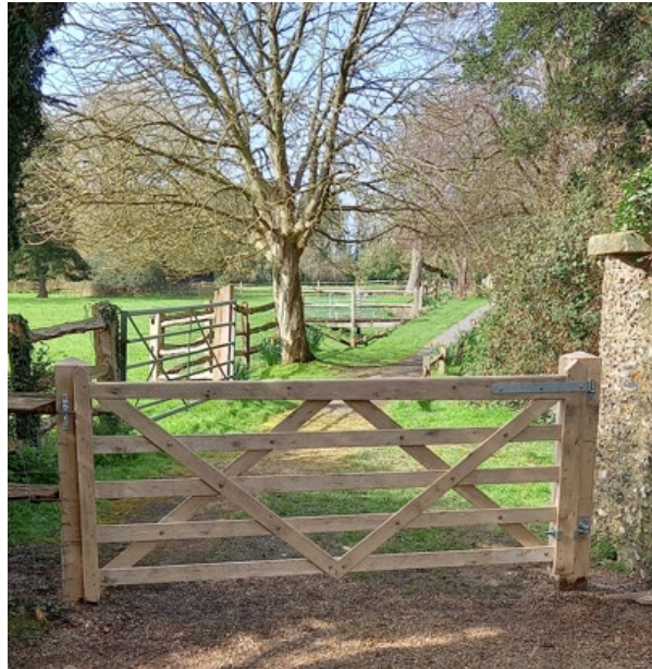
Image 10 New gate for a church in Poling
