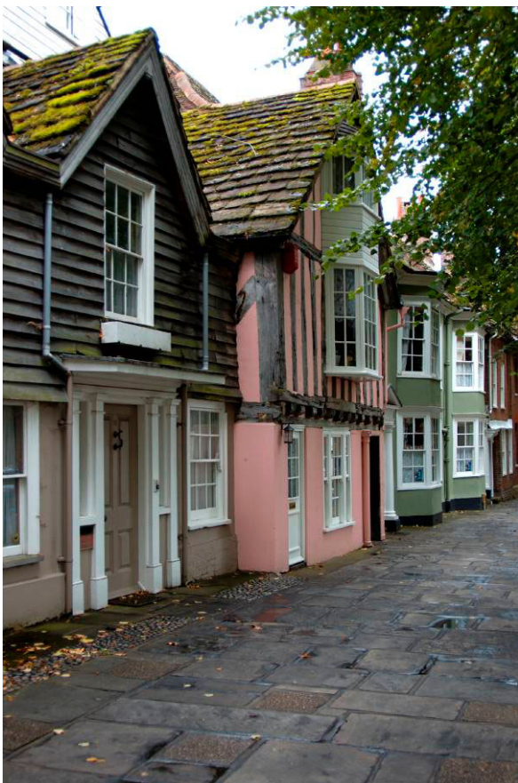
Fig. 14. 11-12 Causeway, showing the exposed 15 th -century timber framing of the cross-wing.
