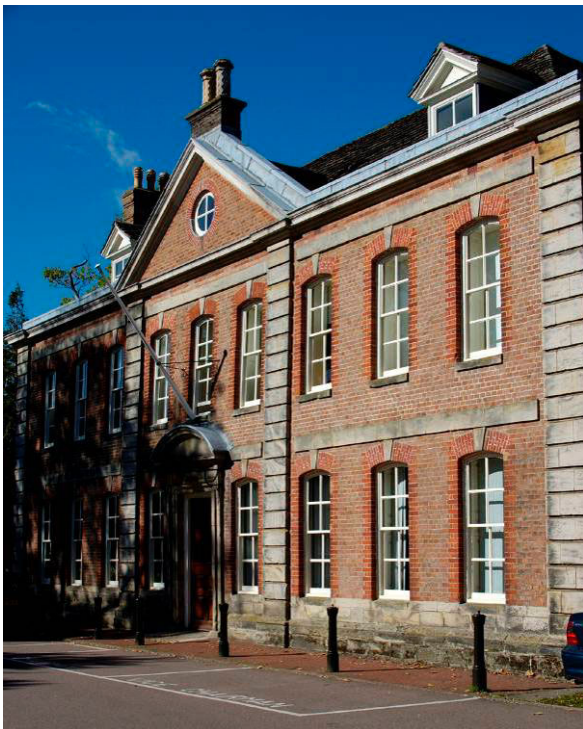
Fig. 17. Horsham Park house: early 18 th -century south-east front.
