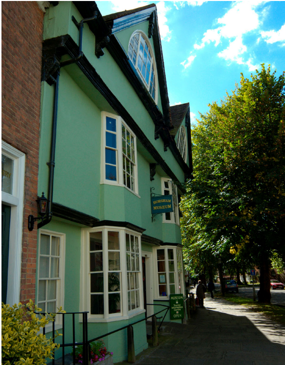
Fig. 19. Causeway House (9 Causeway), home of Horsham Museum: c.1600 timber-frame frontage to medieval house behind, possibly representing post-medieval encroachment.
