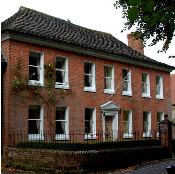
Fig. 18. The Chantry, 27 Causeway: the 18 th -century façade hides the medieval timber frame (of a barn) behind.
