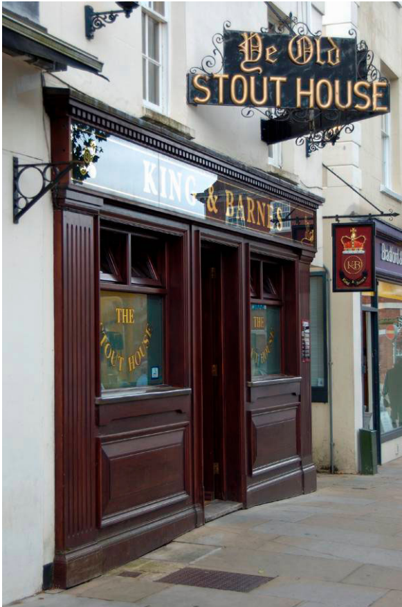
Fig. 6. The Old Stout House, 29 Carfax: the King & Barnes pub façade hides a 16 th -century timber-framed building.
