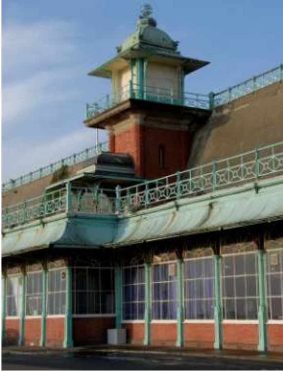
Fig. 14. Madeira Terrace, with lift opposite Marine Square.
