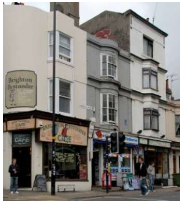
Fig. 55. Terminus Road (1840s): Regency-style bow windows and canted bay windows on modest terraces.
