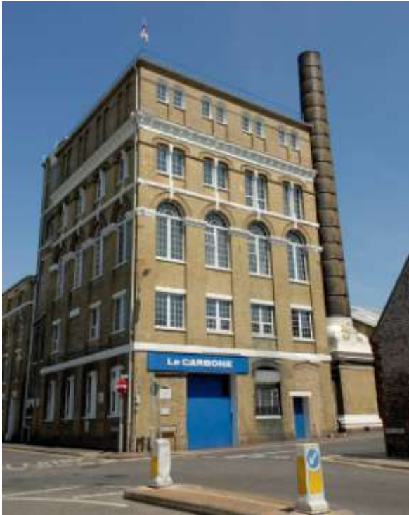
Fig. 60. Former Southdown Brewery, Portslade (1881).
