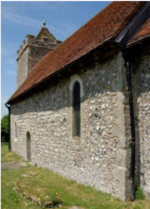
Fig. 29. St Helen's, Hangleton: south wall of nave.
