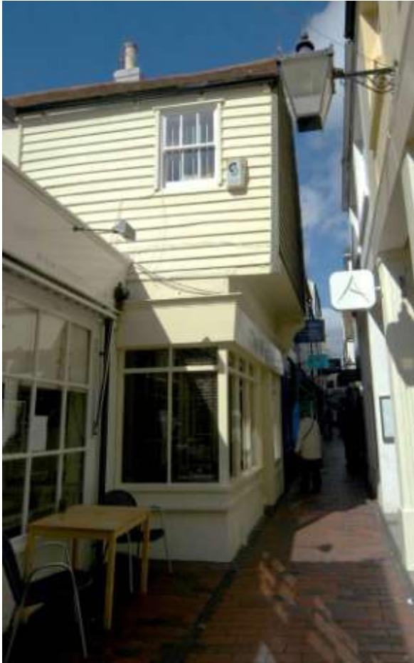
Fig. 37. Timber-framed construction at 43 Meeting House Lane (probably 18 th -century).
