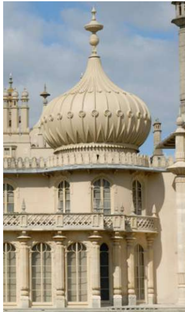
Fig. 40. The Royal Pavilion: detail of east elevation showing bow window by Henry Holland (1786-8) surviving under Nash's largely cosmetic remodelling of 1815-22.
