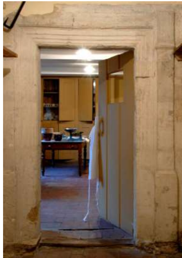
Fig. 45. Preston Manor: late 16 th -century doorway (previously external) to basement kitchen.
