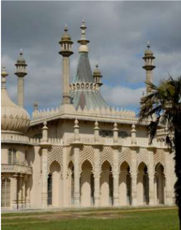
Fig. 9. The Royal Pavilion: east elevation of the Music Room, from the remodelling of 1815-22, by John Nash.
