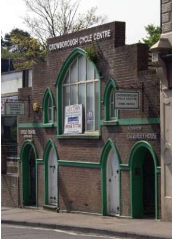
Fig. 7. Former Congregational (later Strict Baptist) chapel, the Broadway (1896): the original gable has been removed.
