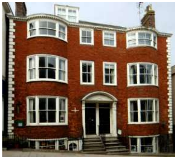
Fig. 33. 199 and 200 High Street (School Hill): late 18 th -century mathematical tiles and wooden quoins.
