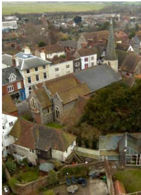
Fig. 22. St Michael's church, High Street.
