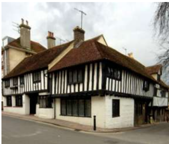
Fig. 31. 49, 50 and 51 Southover High Street.
