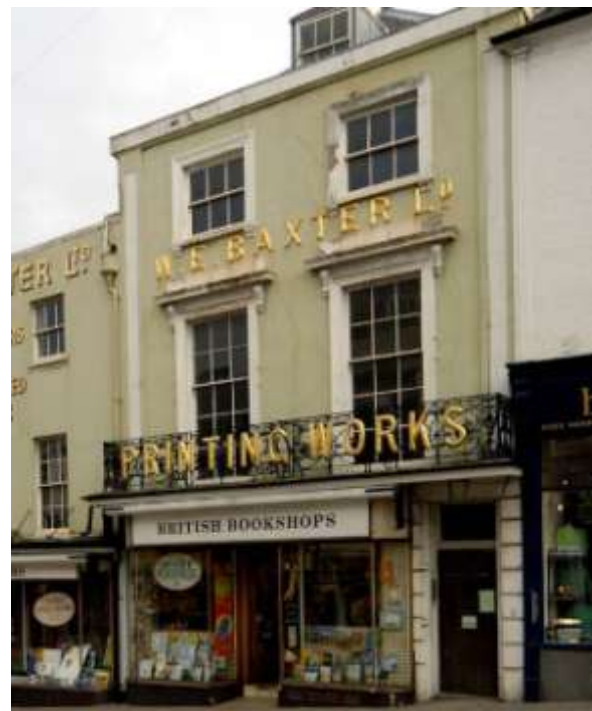
Fig. 38. 34 High Street (School Hill): early 19 th -century stucco refacing of 16 th -century timber-framed townhouse.
