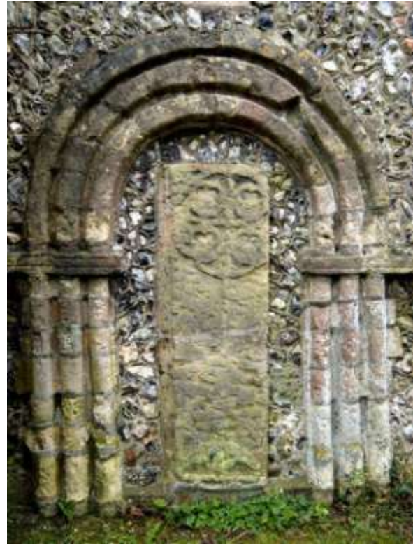
Fig. 3. St John-sub-Castro: 11 th -century former south doorway, re-sited in the 19 th -century church.
