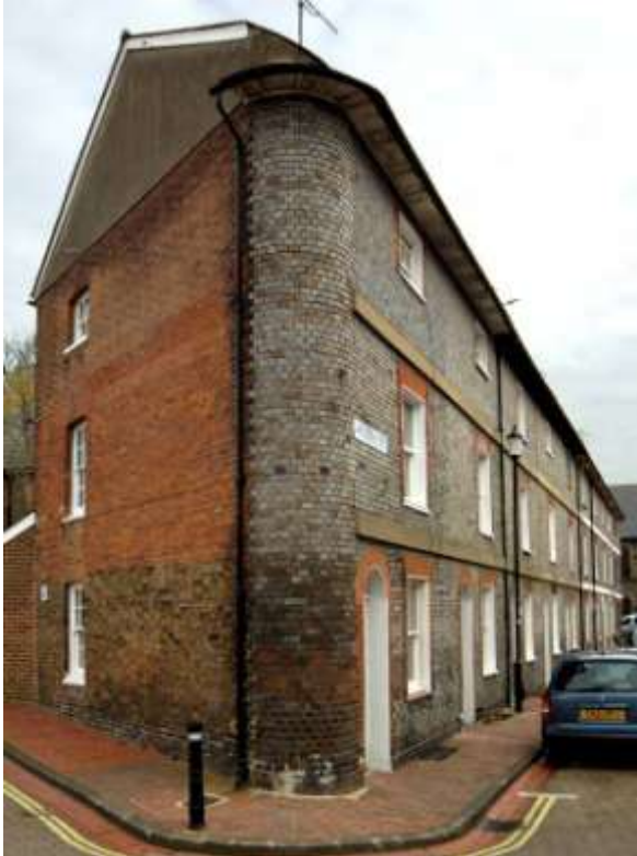
Fig. 37. Waterloo Place: early 19 th -century terrace with brick façade to flint-rubble walling.
