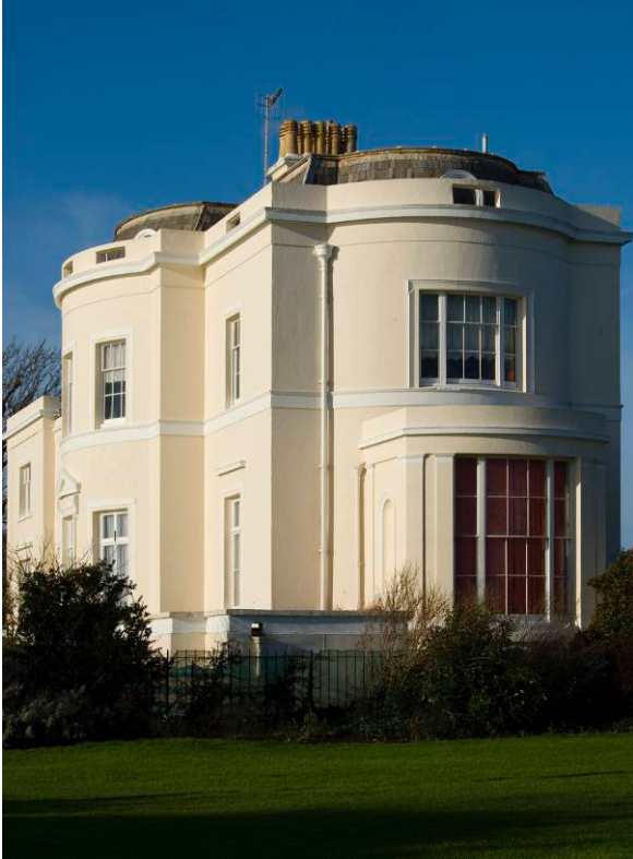
Fig. 26. Beach House, Brighton Road.
