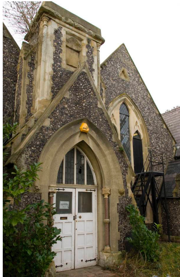
Fig. 13. Former Christ Church school, Portland Road.
