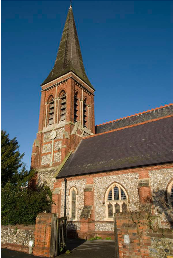
Fig. 30. St Botolph's church, Lansdowne Road, Heene.
