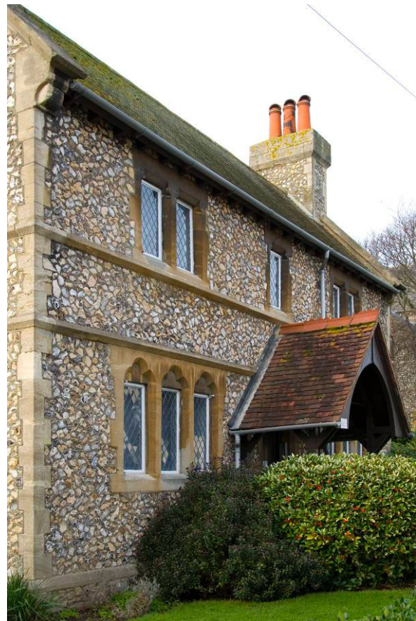
Fig. 29. Humphries Almshouses, Portland Road (1867).
